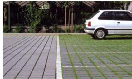
Permeable surfaces allow for groundwater recharge and reduce stormwater runoff.
